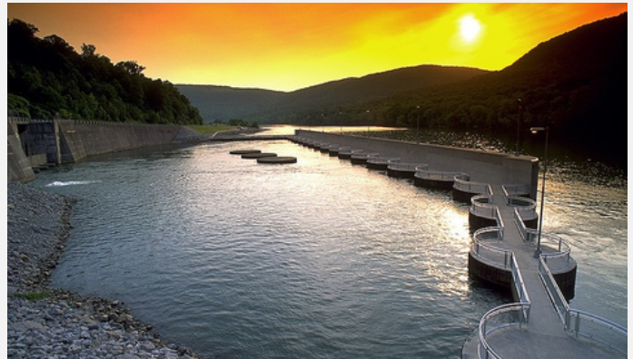
Raccoon Mountain Pumped Storage Plant, photo credit Tennessee Valley Authority
