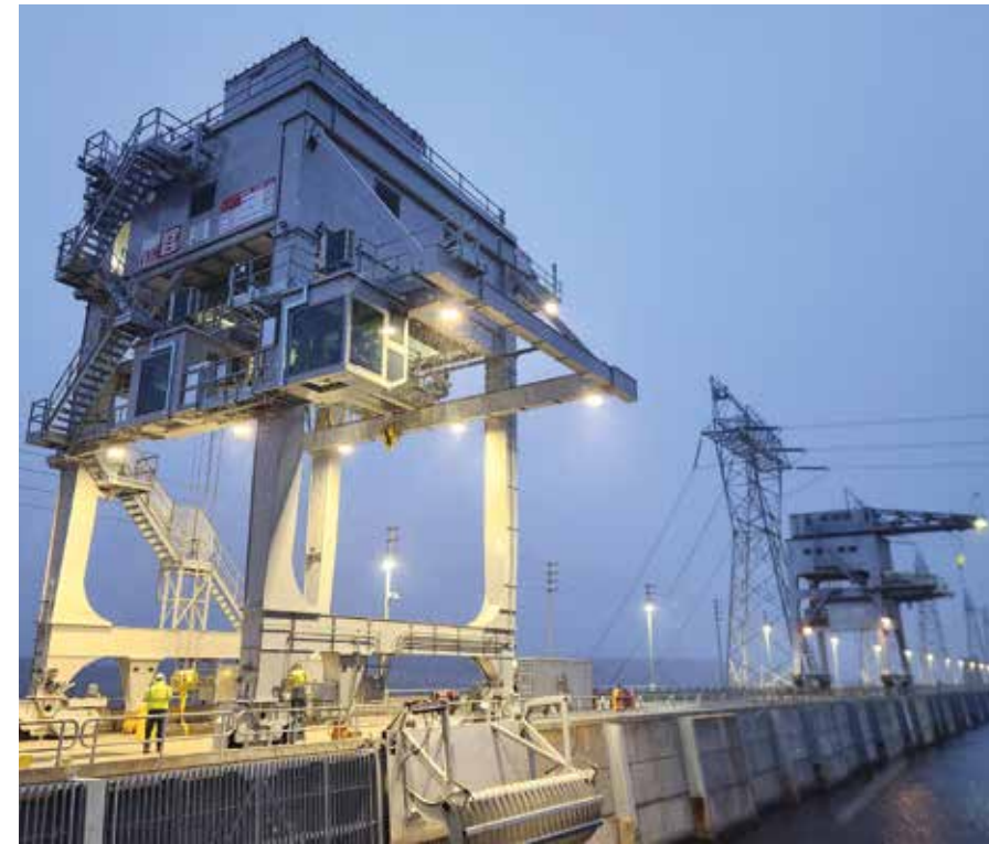
New water intake gantry crane with the old one behind
