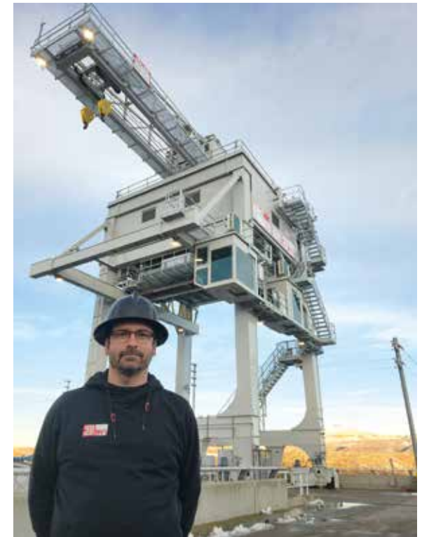
Louis-Philippe, site supervisor, in front of the water intake gantry crane
