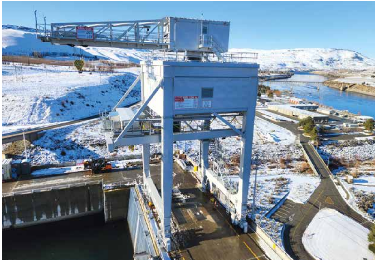
Water intake gantry crane stationed at the end of the dam
