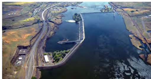
Figure 5: The Dalles Dam on the Columbia River.
