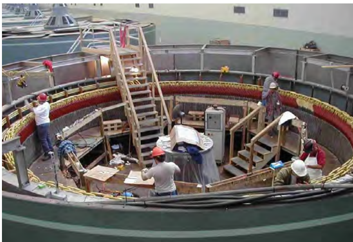
Figure 3: Generator Rewind.
