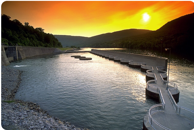
Raccoon Mountain Pumped Storage Plant. Source: Tennessee Valley Authority (TVA)
